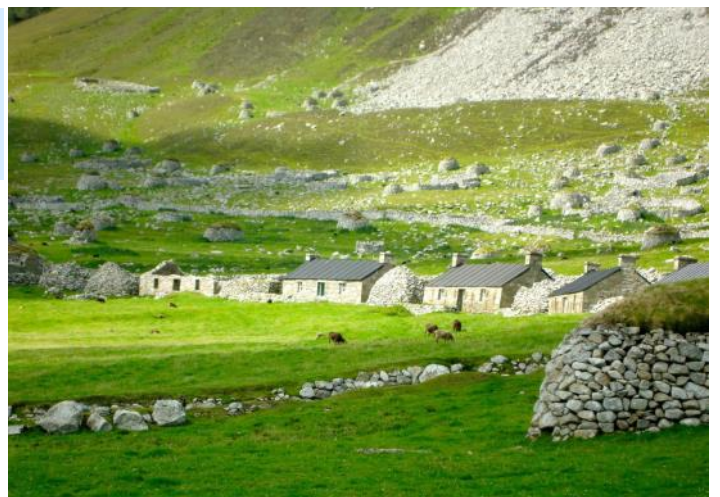
The restored St kilda cottages in Village Bay on the main island of Hirta surrounded by the unique stone cleit structures that the St. Kildan's used to store and dry out many of the birds caught during the summer months to see them through the hard winter conditions.
