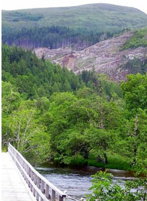
Works above Caig Falls from a distance
