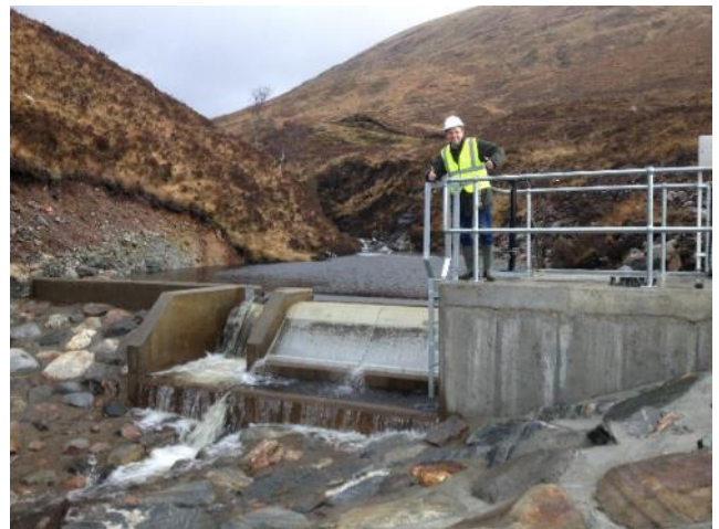
Donald Andrew Cameron at one of the hydro schemes up Loch Arkaig side already generating and sending power to the grid.
