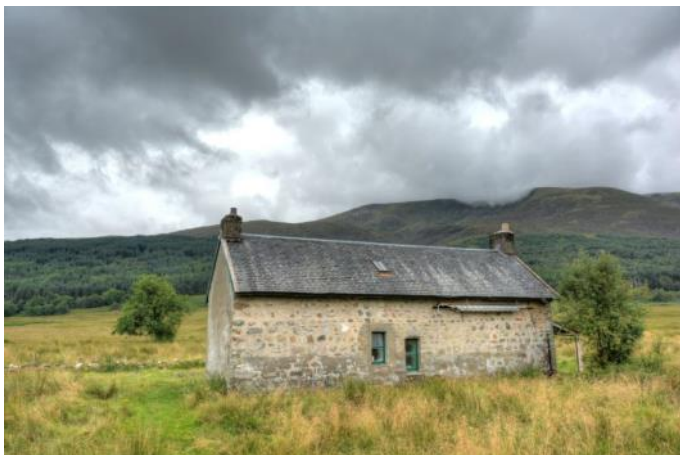
Photograph 7: Another view to the SSW showing the northern face of the bothy (now maintained by the volunteer work of bushwalking clubs). My main point here is that the bothy's 240 year stone-work is still robust
