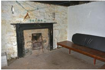
Photograph 9: Room 2. Here the fireplace has, at some stage in the past, been reduced in size. I am left wondering which room was the original kitchen and dining area?
