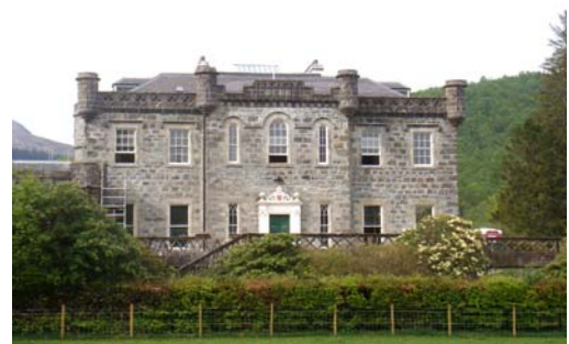
Achnacarry after removal of scaffolding revealing the renovated roof.
