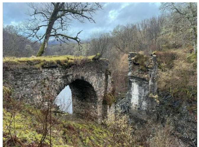
The remains of High Bridge by the Spean
