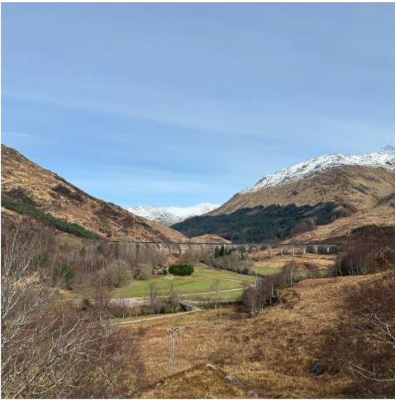
The Glenfinnan Viaduct
